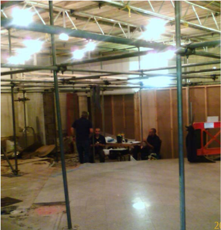
Centre City Lobby Under Construction
