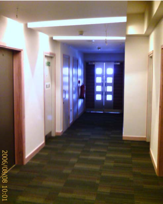
Lighting to be Completed
