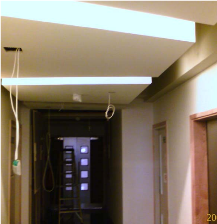
7th Floor Lighting to be completed
