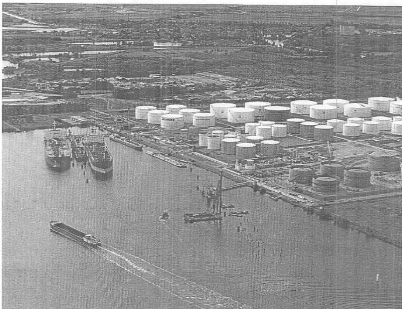
Oil tanking Amsterdam, with new tanks going up
