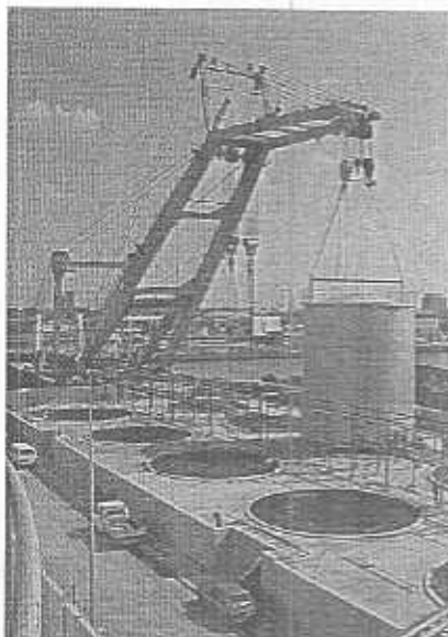
Tanks going in at LBC Antwerp
