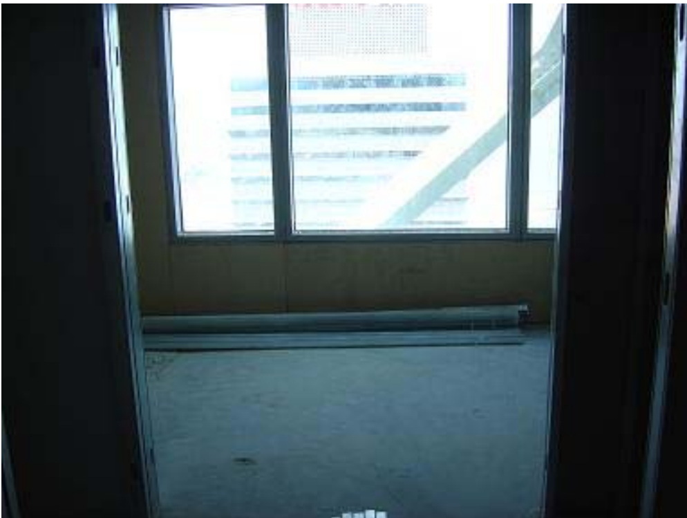
Showers under construction
