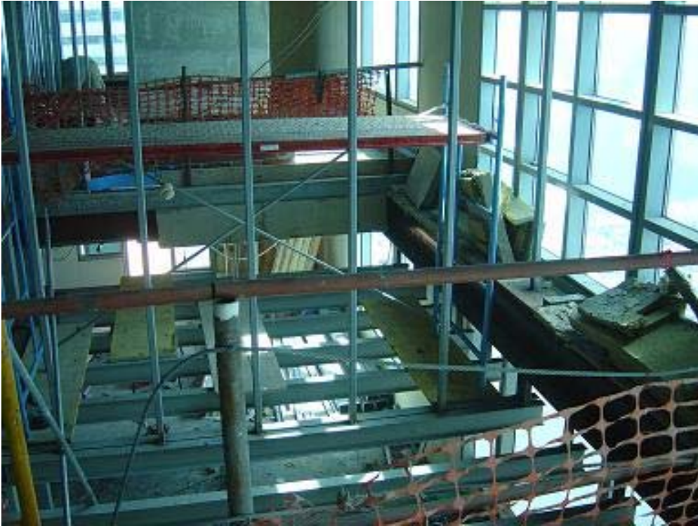
New Pool Slab under construction
