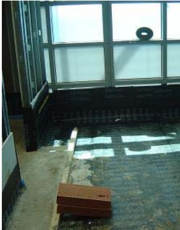
Sauna & Steam Room under construction
